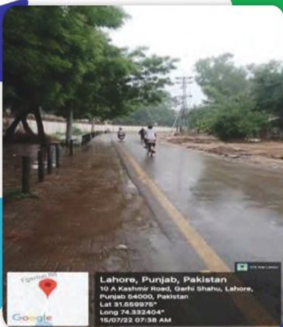
Fig 21: View of Kashmir Road after the construction of Stormwater Storage Tank
