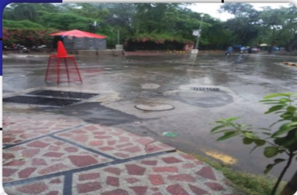
Fig 19: View of Lawrence Road after the construction of Stormwater Storage Tank
