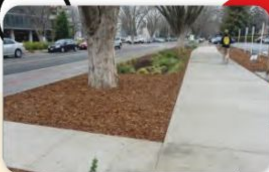
Green Streets with Infiltration swales
