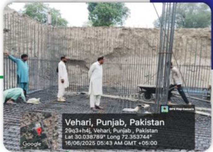
Fig 17: Under construction Stormwater Storage Tank at Gol Chowk, Vehari
