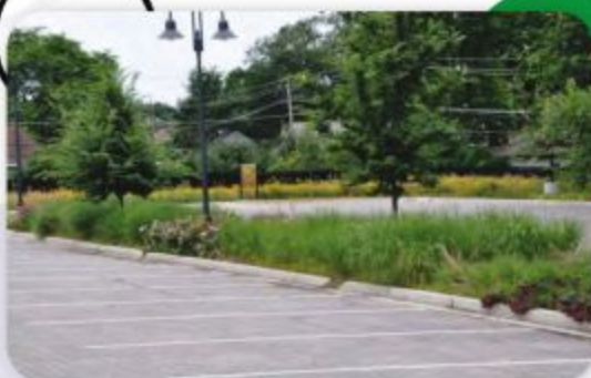
Permeable paving Drains used in vegetated swale used in Parking lot, Elmhurst, Illinois, USA
