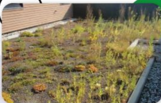
Green Roof in Villa Park, Illinois, USA
