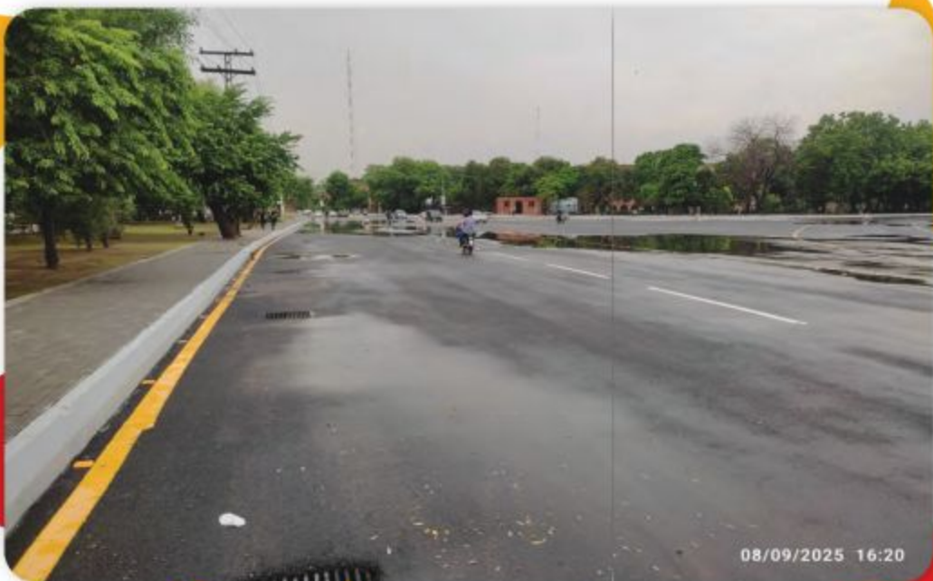
Fig 25: View of Nishter Park Stadium Complex Road after the construction of Stormwater Storage Tank
