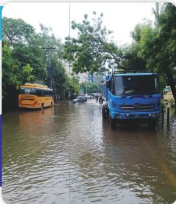
Fig 20: Accumulation of Rainwater on Kashmir Road before the construction of Stormwater Storage Tank
