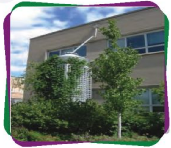
Rainwater capturing from Roof Top
