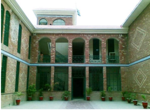
Figure 14: Front view of MC Office Building
