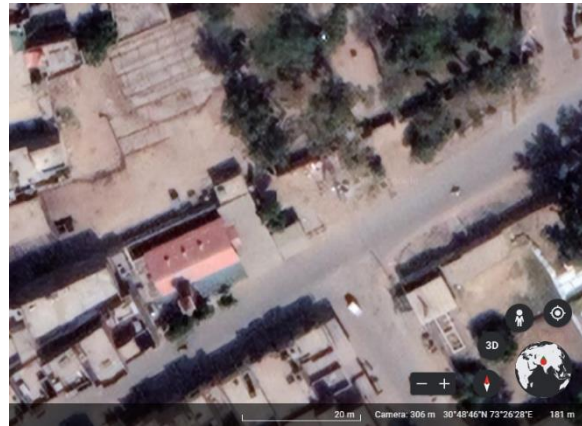
Figure 16: Aerial view of Slaughter House
