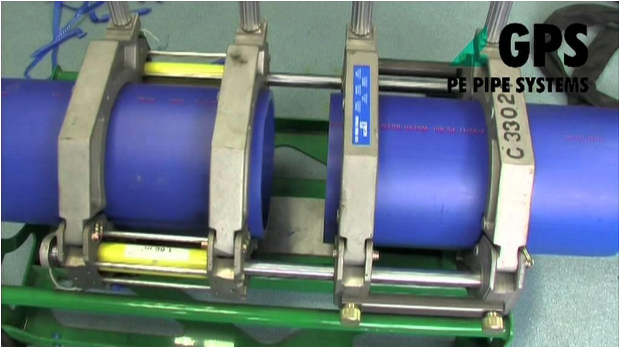
Figure 4-4 Aligning the HDPE pipe for welding
