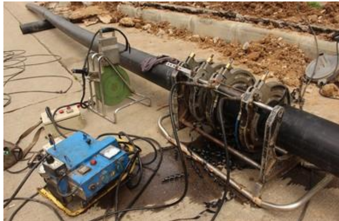
Figure 4-6 Heating of surface with heater for welding of HDPE pipe
