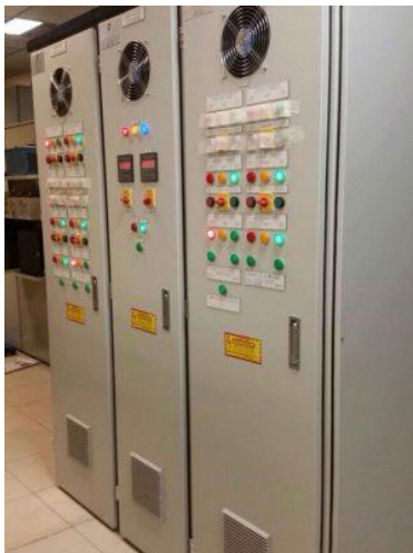
Figure 4-42 Motor starter and breaker
