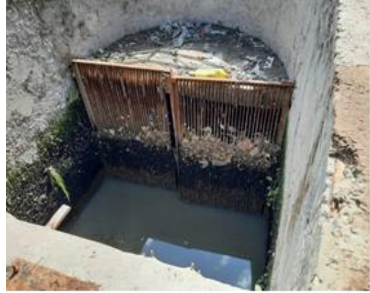
Figure 4-19 Bar screen and a choked impeller
