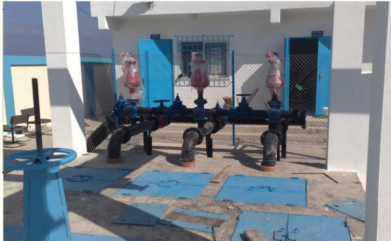
Figure 4-7 Force main and header
