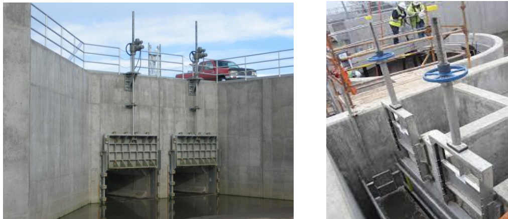
Figure 4-22 Penstock gates
