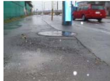
manhole damaged
