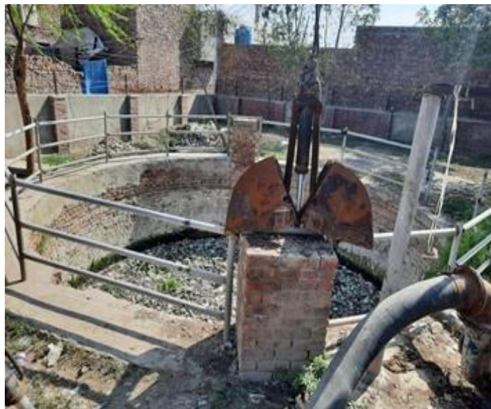
Figure 4-20 Cleaning of wet well with clamshell excavator
