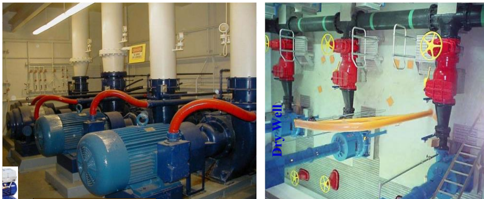
Figure 4-6 Inside and outside dry well or pump house 23
