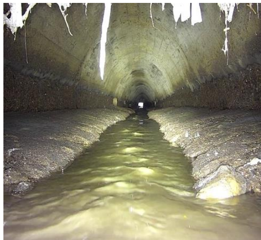
Figure 2-2 Sewer inspection with camera
