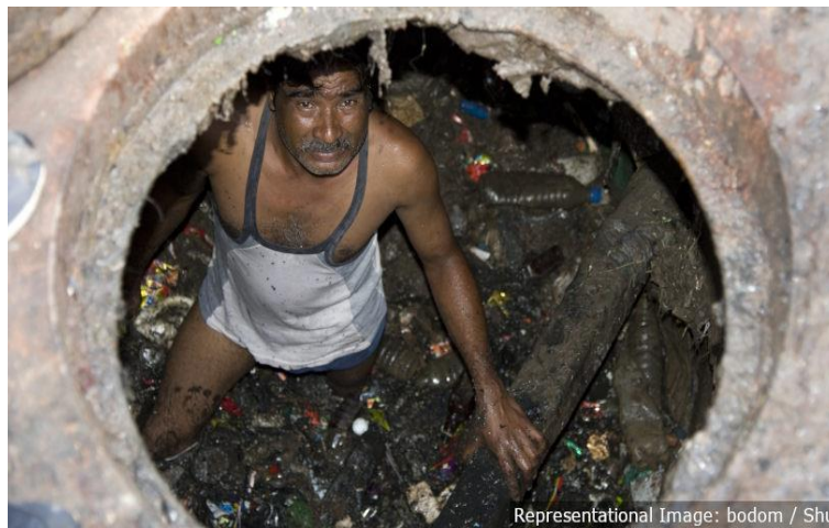
Figure 1-10 Solid waste dumping in the sewer
