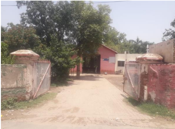
Figure 21: Front view of Fire Brigade
