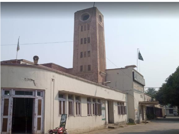
Figure 14: Front view of MC Office Building
