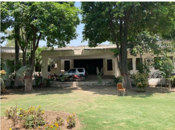
Figure 13: Front View of Main MC Building
