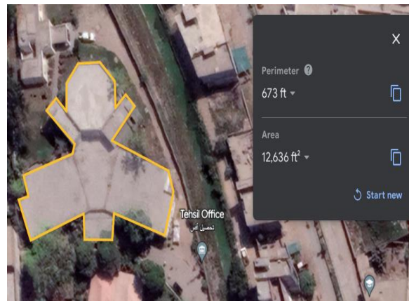
Figure 16: Top View of Main MC Office building-Offices Block
