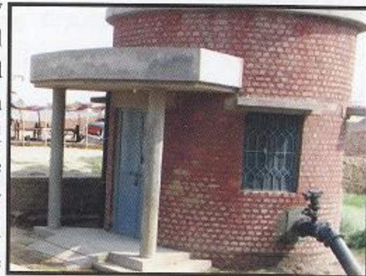
Water Works at TMA Kasur
