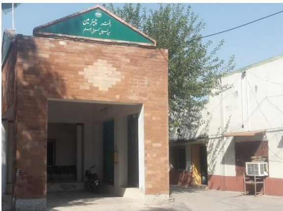
Figure 14: Front View Of Main MC Office Building
