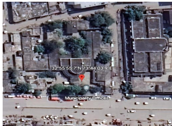
Figure 15: Aerial View of MC Office Main building
