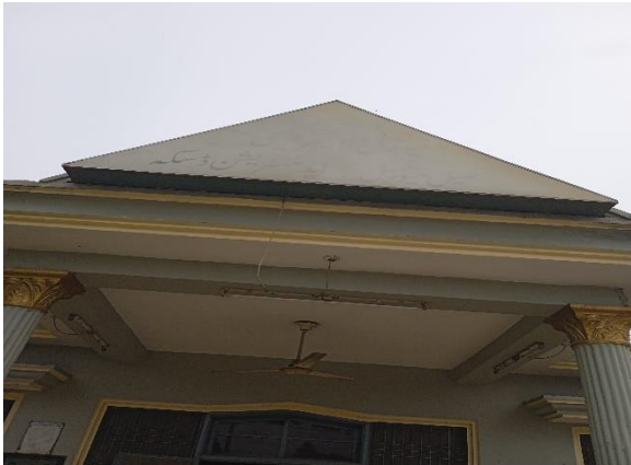
Figure 20: Front view of the Library
