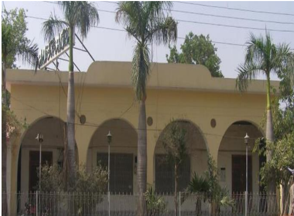
Figure 16: Front view of Mc Office No.2
