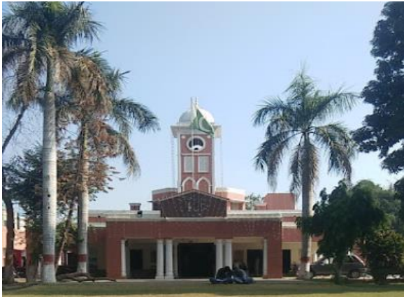
Figure 14: Front view of MC Office Building
