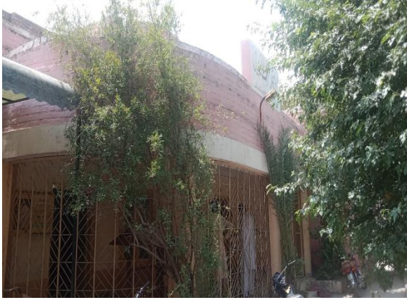
Figure 26: Front view of Library
