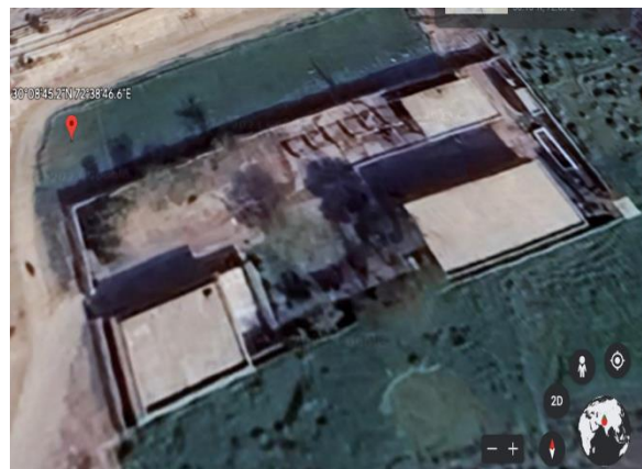
Figure 29: Aerial view of Slaughter House
