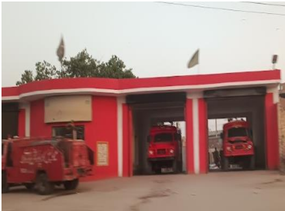
Figure 23:Front view of Fire Brigade
