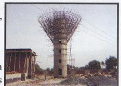
Visit to Liaquatpur - Water Supply System
